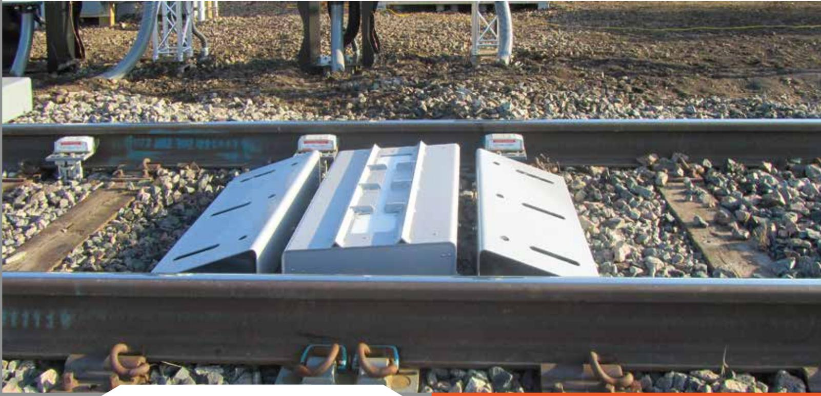
CouplerView-Pin is an automatic wayside detection system that is designed to detect defects in the F-type coupler securement mechanism. For F-type couplers, the system inspects the coupler vertical pin carrier plate or pins and the corresponding fasteners.
